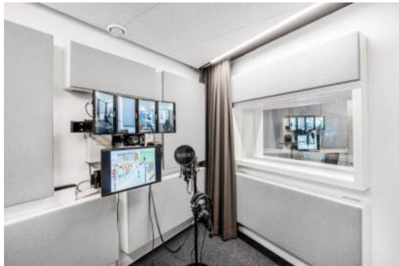
The speech lab has five acoustically treated recording booths. It is possible to record a participant in each booth simultaneously allowing for directed speech experiments with up to 5 participants. Each booth is equipped with a Røde 1000 large diaphragm condenser microphone and DT 770 head phones. Alternatively there are also DT250 headsets.
